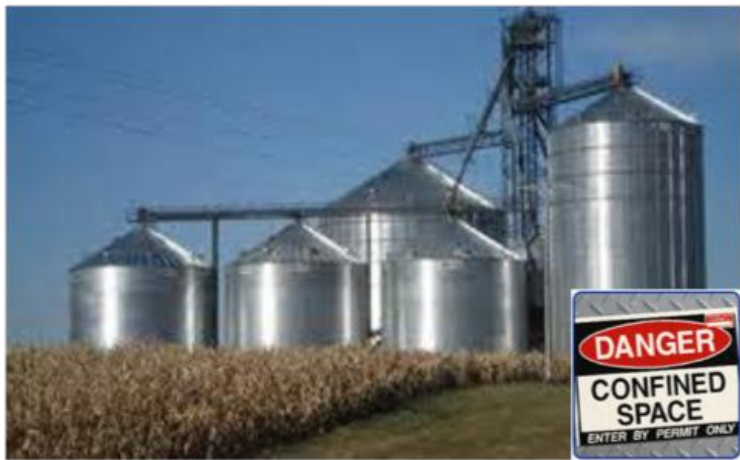
Figure 1. Grain bins are excellent tools for storing and marketing grain, but can also pose a significant safety hazard. Knowing the safety rules and adding proper signage around bins can help prevent tragedies.
